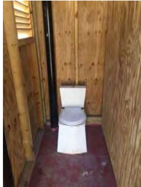
Left: One of the VIDP's in Naggo Head community; middle up: receptacle in Naggo Head Rd; middle down: Concrete plate to seal dry tank for later use; right: inside view of VIDP (dry toilet and vent pipe).
