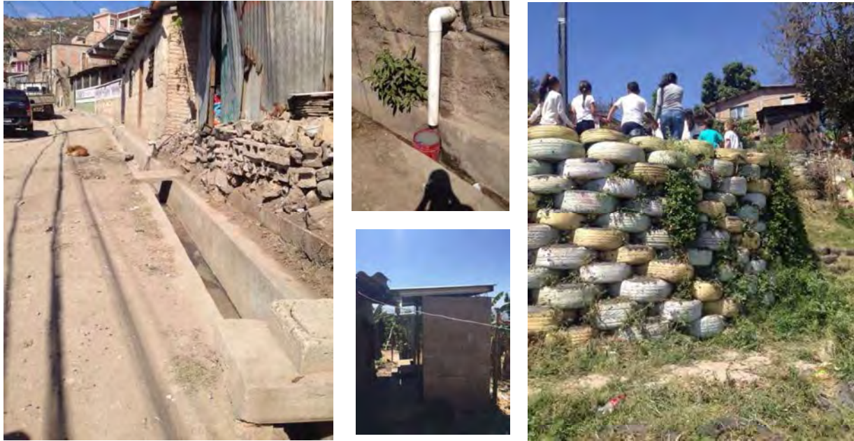
Left: drainage ditch constructed in José Arturo Duarte community; middle up: recollecting gray water for reuse; middle down: sanitation modules; right: communal park (with recycled tires).
